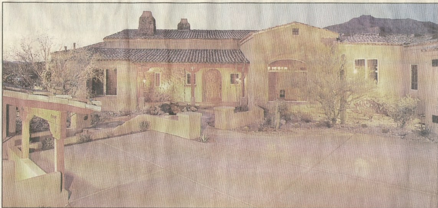
Dan Boylan uses salvaged wood from train trestles, dismantled granaries and old buildings to add historic accents to the custom homes he builds in Gold Canyon.
